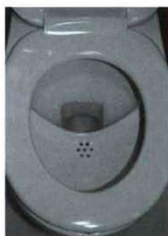
Figure 4. The bowl of the separate drain-off (separating) toilet (Novaquatis)
