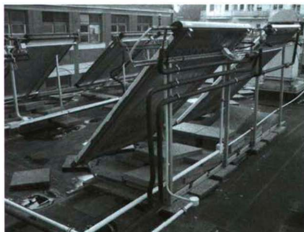
Figure 4. Measuring system with Buderus collectors
