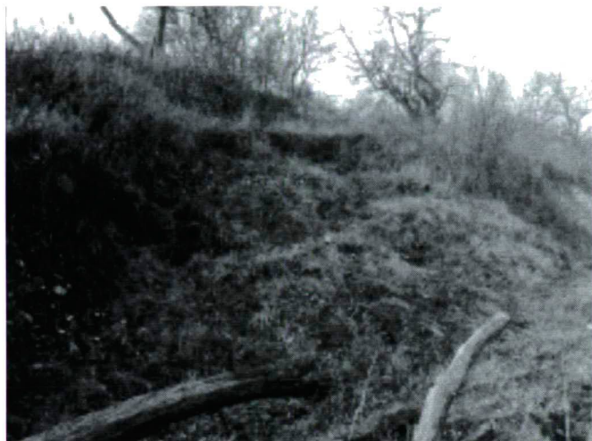
Fig. 3. Front of a landslide in József Attila residential area.
