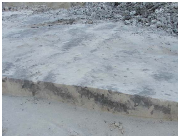
Fig. 9 Plough marks stretching from north to south (foto: Szabolcs Rosta)
